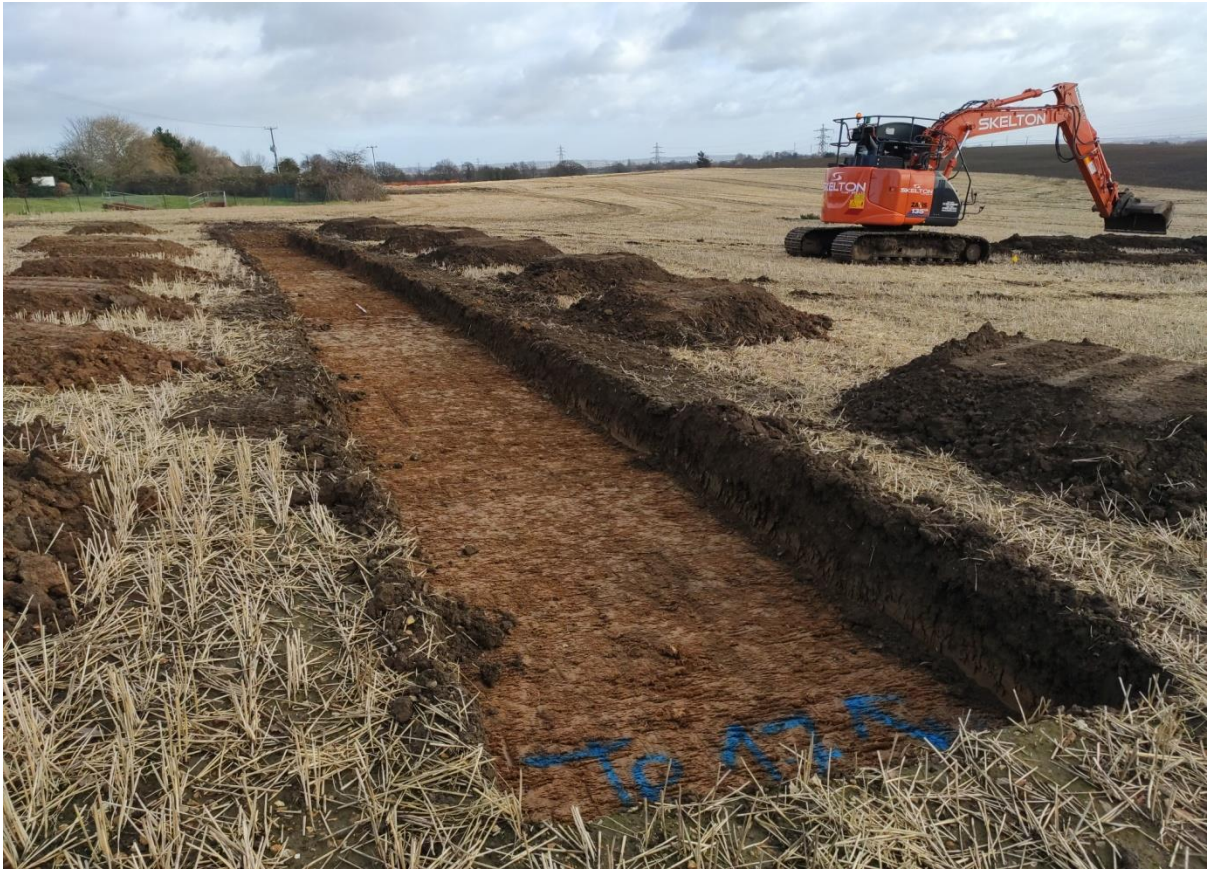
Plate 17: Trench 17, looking NE with one-metre scale.
