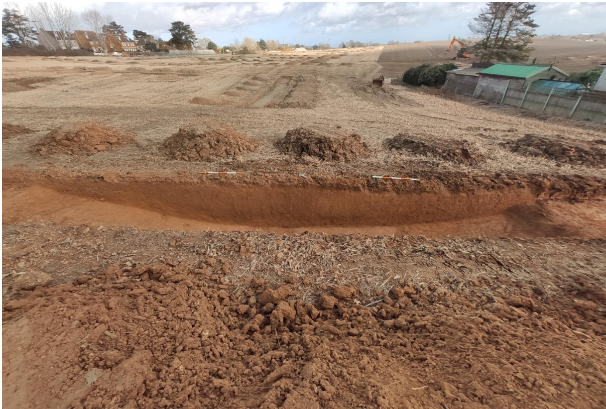
Plate 1: Showing the site and Drove way (Holloway) [106]. Looking NE with two one-metre scales.
